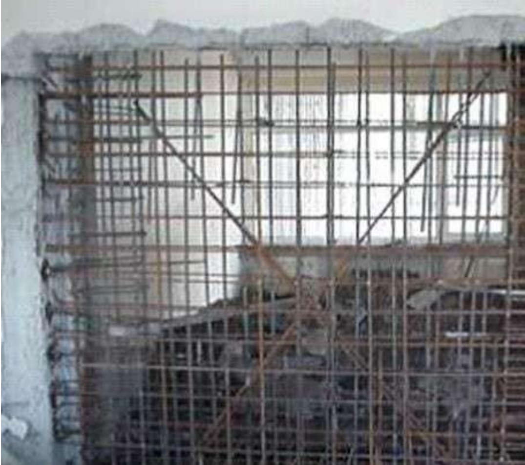
Fig 2: Additional Shear Wall
